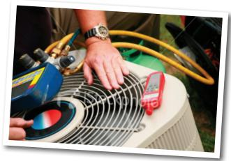
These routine maintenance procedures are important because dirty air conditioning coils make it difficult for the equipment to properly cool your home. To compensate, your air conditioning unit may run longer, increasing energy costs and reducing the life of the equipment. Cleaning your equipment ensures that it will work efficiently, as airflow problems can reduce efficiency by up to 30 percent.
