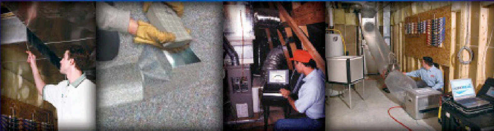
AeroSeal technician conducts initial diagnosis by analyzing airflow. MW registers are covered in order for air to escape only through leaks. A professional AeroSeal technician will monitor the duct leakage in your home. AeroSeal software allows the technician to accurately measure the duct leakage in your home.
