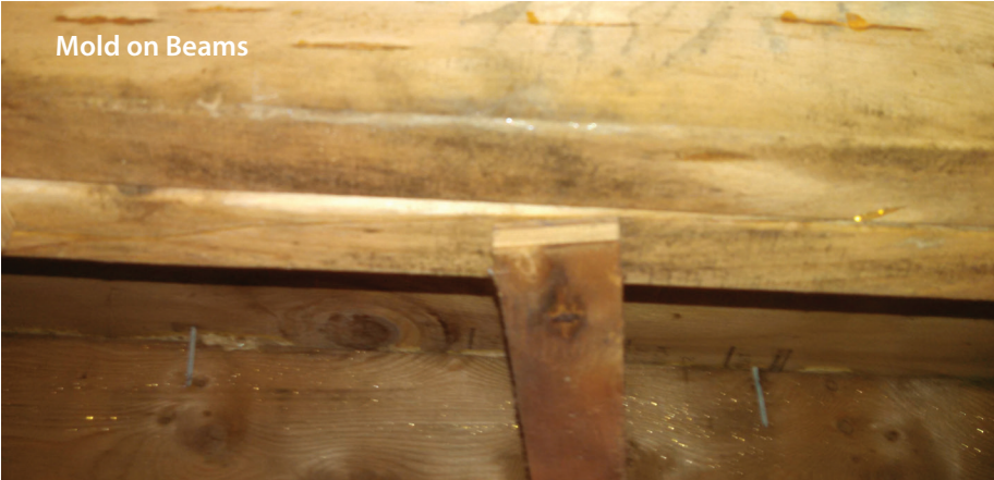
Crawl Space Before
