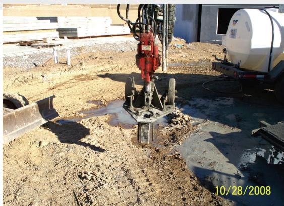
The solution proposed by Foundation Specialties and James L Burke, P.E. was the use of hollow bar micropiles drilled and grouted through the boulder fill material and into bedrock to support the footing. ECP was contacted to provide under-footing brackets that would connect the micropiles to the footing and transfer the loads to the micropiles..
