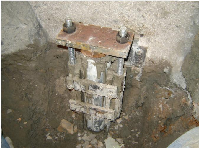
After the micropile grout achieved the design compressive strength of 4000psi, the micropiles were loaded to 17 kips and locked off in the brackets. This transferred 90% of the wall load to the micropiles. The gap between the wall panels and the footing was filled with grout to completely transfer the load to the micropiles
