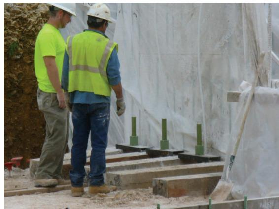
Ground anchors are used to control strong uplift forces by providing an active post tensioned downward pull on a structure. One of the most common uses of these anchors are bridge abutments. Bridges have high rotational or eccentric forces on the abutments which are counter-acted by the down pull of the tensioned anchors.
