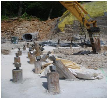
Micropiles are a small diameter replacement pile capable of supporting compression, tension, and lateral loading. The load capacity of the micropile is generated by the large cross-sectional area of reinforcing steel and transfer of the loads to the surrounding material via the ground grout bond. This load transfer mechanism allows micropiles to be used in geologic conditions that would
