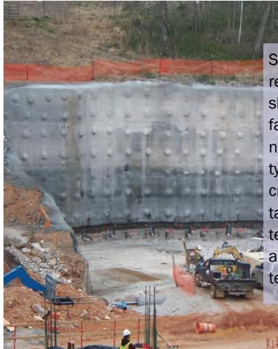
Soil nails are fully grouted steel reinforcing rods drilled into a slope designed to penetrate a failure plane and retain the nailed materials. The nails are typically covered with a shotcrete retaining wall. These retaining structures can be either temporary or permanent. An anchored earth retention system is very similar to a soil nail
