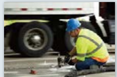
Traffic lanes remained open during installation
