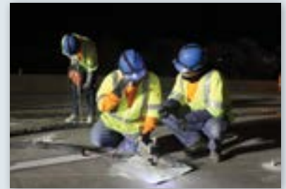
PolyLevel being injected in liquid form
