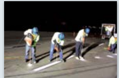
5/8 inch injection holes drilled in to road slab
