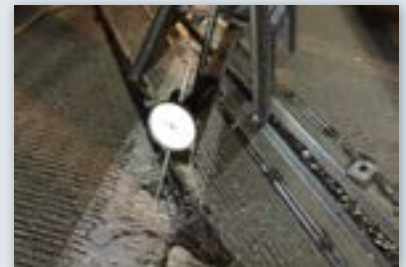
Slab movement precisely monitored with dial gauges
