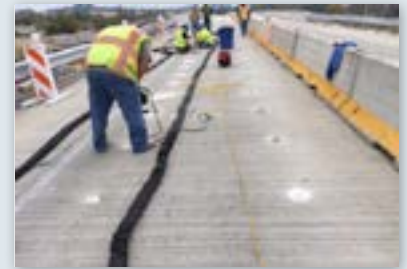
Injection holes being drilled
