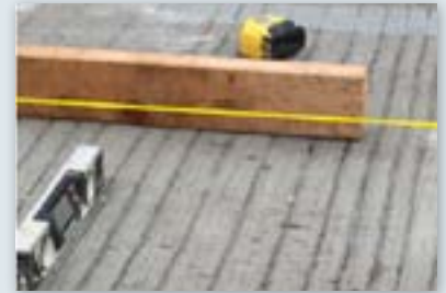
String line shows the extent of the slab settlement
