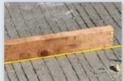
String line shows slab returned to a level position
