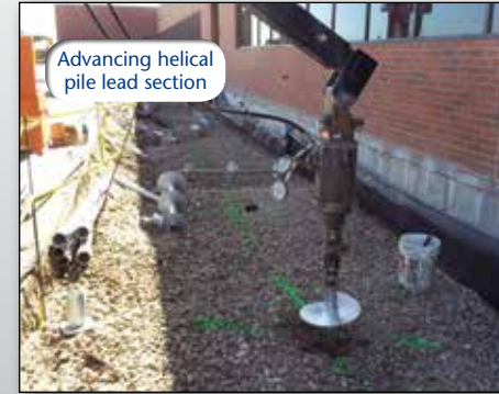
Pile installation close to building
