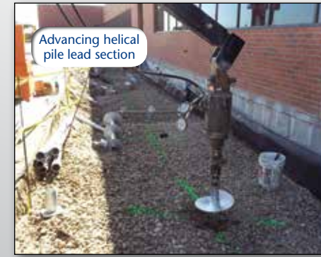
Pile installation close to building
