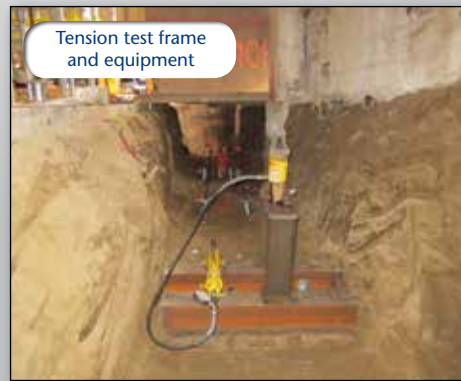
Installing vertical pile; equipment between temporary supports
