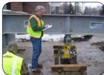
Don Deardorff (FSI) assisting with a helical pile load test.
