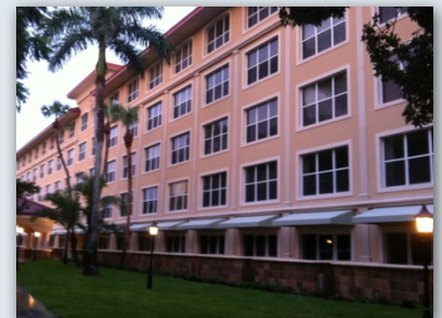
Westminster Manor after renovation
