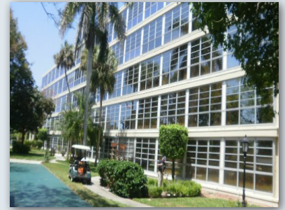
Westminster Manor before renovation
