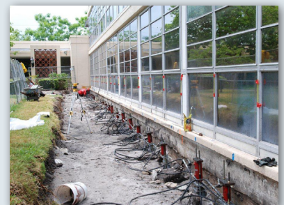
Uniform seating load applied to the piers
