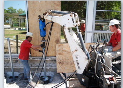
Advancing helical piers next to prepared/notched footing
