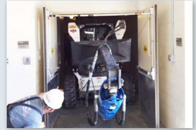
Maneuvering skid steer through standard double doorway
