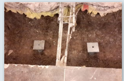
Piles installed and fitted with new construction caps
