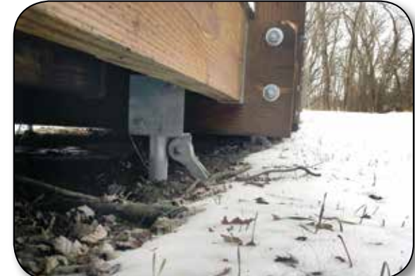
Custom saddle bracket connected with clevis to battered helical pile.
