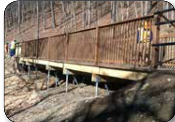
Boardwalk supported on 2.375" O.D. vertical and battered helical piles.
