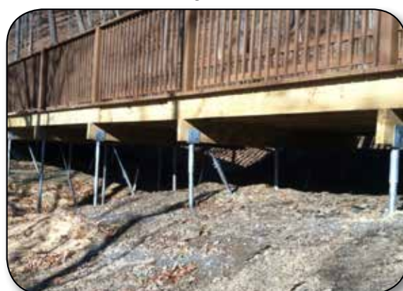
Boardwalk supported on 2.375" O.D. vertical and battered helical piles.
