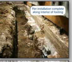
terior and exterior pier installation complete applying uniform load to each pier with hydraulic cylinders
