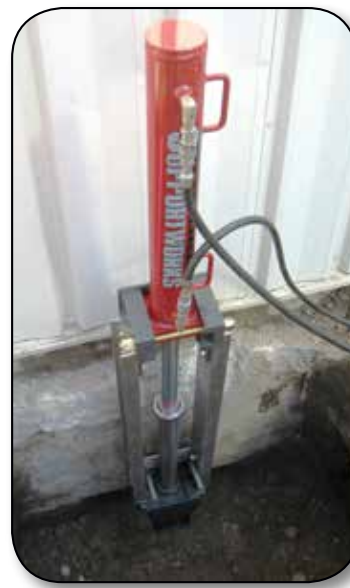
Hydraulic cylinder installing a 2-7/8 inch push pier.
