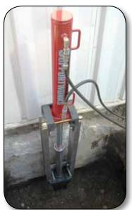
Hydraulic cylinder installing a 2-7/8 inch push pier.
