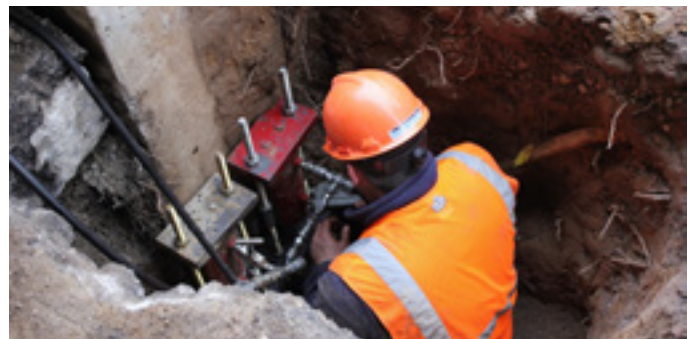
Connecting hydraulic lift cylinders
