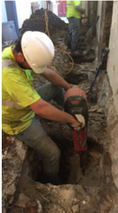
Trimming footing for retrofit bracket placement
