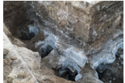
Installed piers at exterior corner
