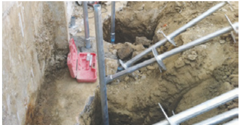
Leads and first extensions staged near installed piles
