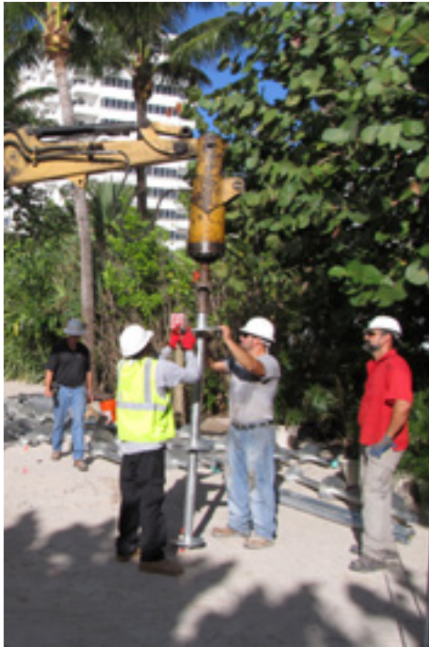
Connecting drive head to helical pile lead section
