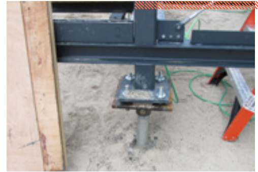
Beach house framing bolted to helical pile
