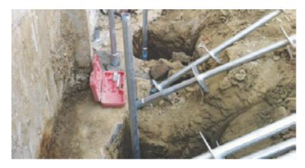
Leads and first extensions staged near installed piles
