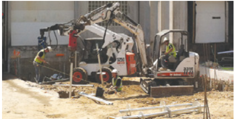
Skid-steer and mini-excavator installing helical piles
