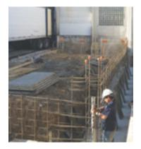
Setting pile elevations within columns and grade beams
