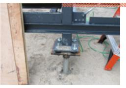
Beach house framing bolted to helical pile
