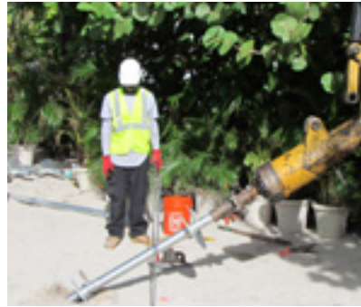
Advancing battered pile
