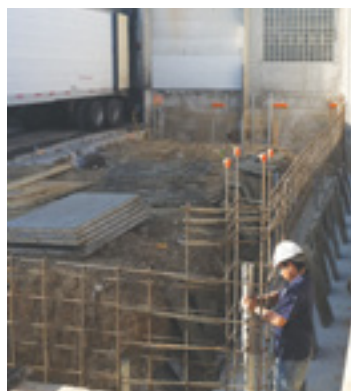
Setting pile elevations within columns and grade beams
