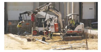
Skid-steer and mini-excavator installing helical piles
