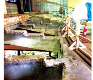
Upper structural slab (left) and lower SOG (right) auditorium seating areas
