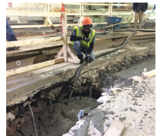
Filling trench with concrete
