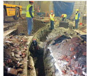
Trench excavation for anchor plates
