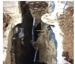
Anchor plates attached to rods and set in excavation
