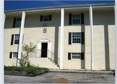
One of the six buildings to be stabilized
