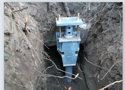
Pier installation complete
