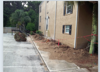
Preparing work area for pier installations
