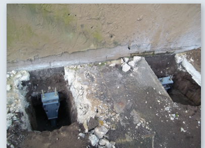
Pier installation complete
