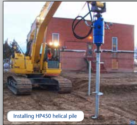
Installing test and reaction piles
