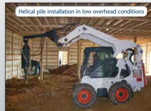
Retrofit pile systems used to re-level structure
