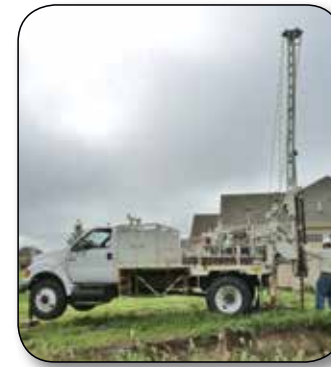
Truck-mounted drill rig
