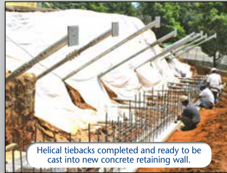
Installation of helical tieback.
