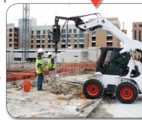
Helical piles to support crane pads at a construction site
