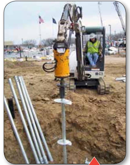
Helical piles to support foundations of a medical center addition
