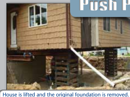
House is lifted and the original foundation is removed.
