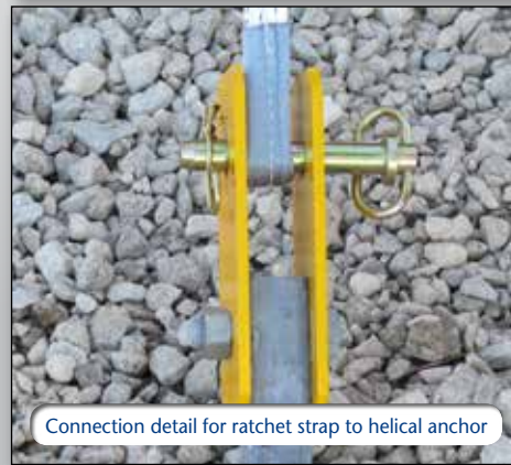
New FSU Flying High Circus tent tied down with helical anchors
