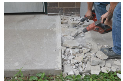
Removing concrete “wedge” prior to installing PolyLevel
