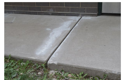
Faulted slab sections returned to original elevation
