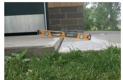
Three inches of differential settlement visible after concrete wedge removed
