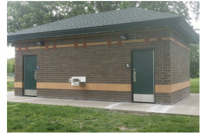
Sidewalk settlement at public restroom
