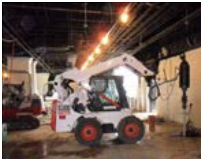
Installing helical piles within basement
