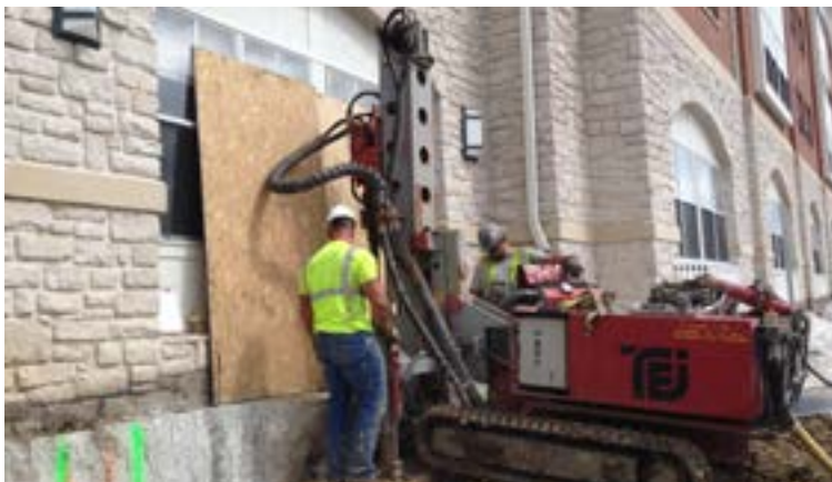
Pre-drilling at production pier location
