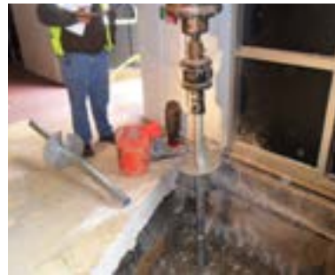
Advancing helical pile
