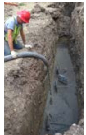
Pouring deadman wall to encase GeoLock® earth anchor plates
