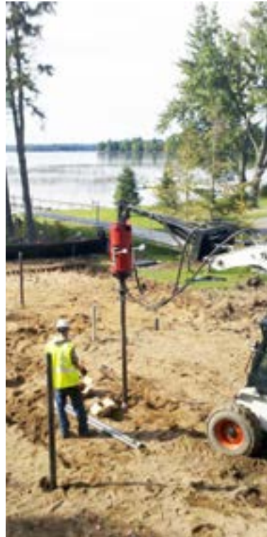
Piles advanced to refusal in deep gravelly sand
