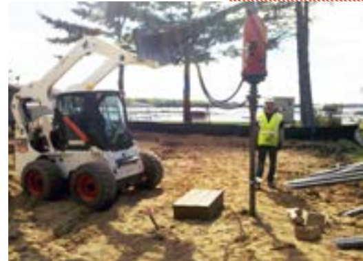
Advancing lead section of 3.5-inch O.D. pile
