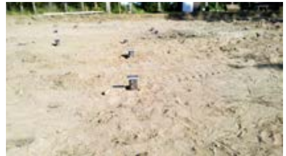
Completed piles and brackets
