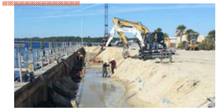
Excavation made behind seawall for tieback installation
