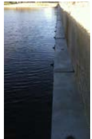
Waler system on stabilized seawall
