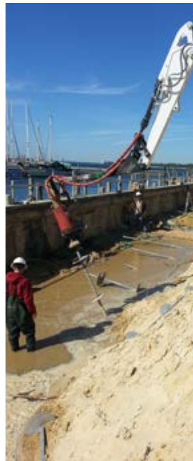
Moving HA175 lead section to position for advancement
