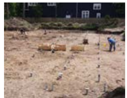
Pile installation complete
