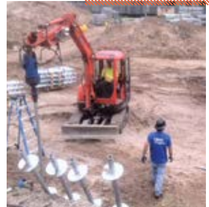
Advancing HP288 helical pile
