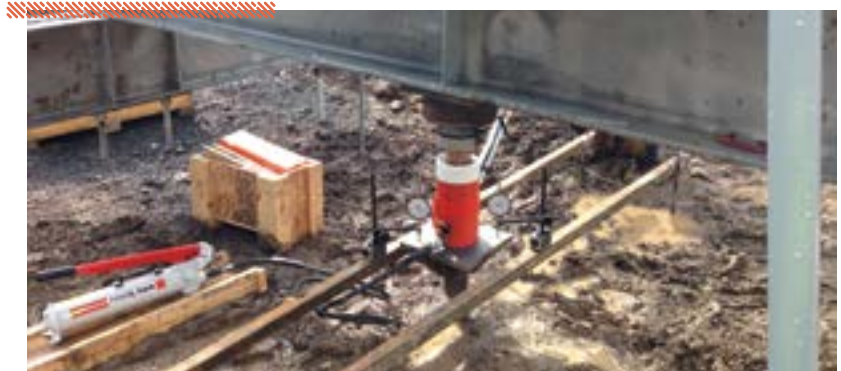
Compression load test
