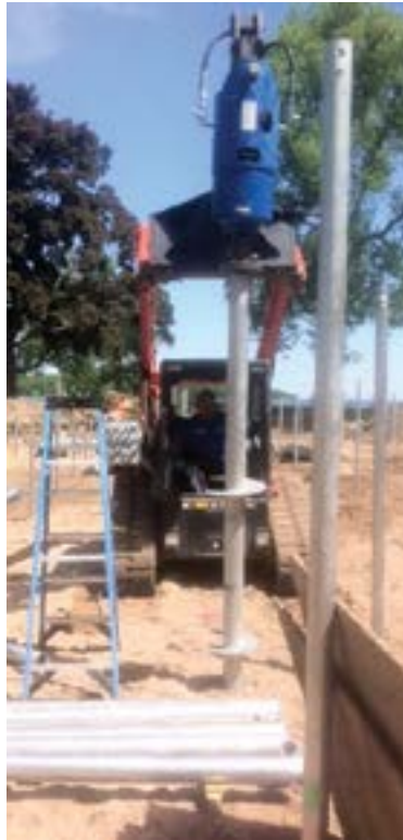
Advancing HP450 helical pile
