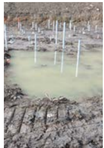
Installed piles
