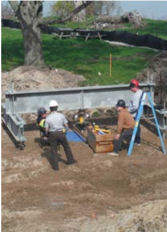
Compression load test
