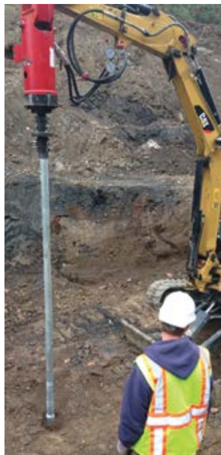
Installing helical pile
