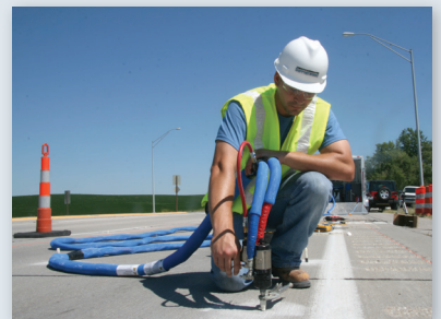
Injecting PolyLEVEL™ and raising slab
