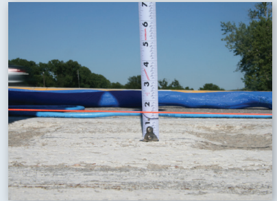
Highway slab before lift
