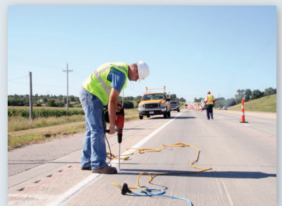
Drilling PolyLEVEL™ injection points
