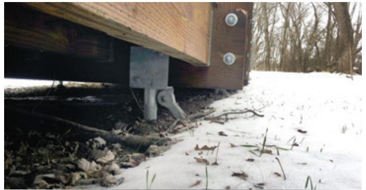
Custom saddle bracket connected with clevis to battered helical pile
