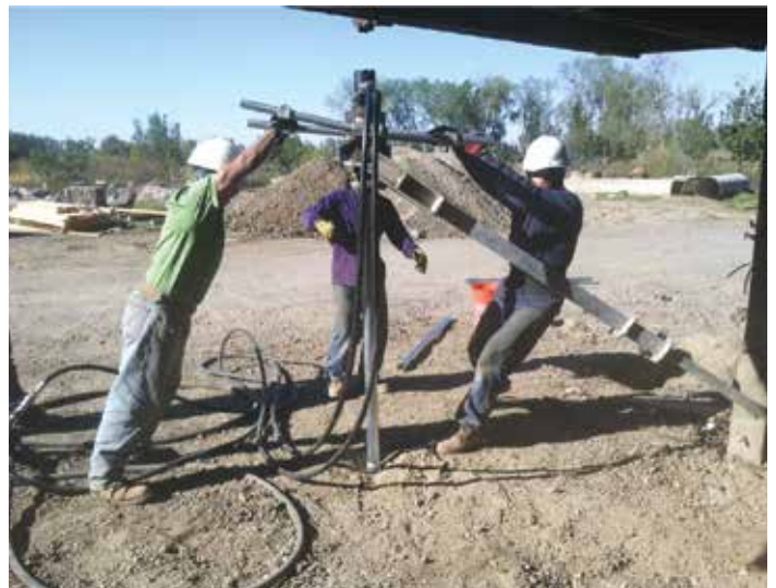
Helical pile installation with hand-held equipment
