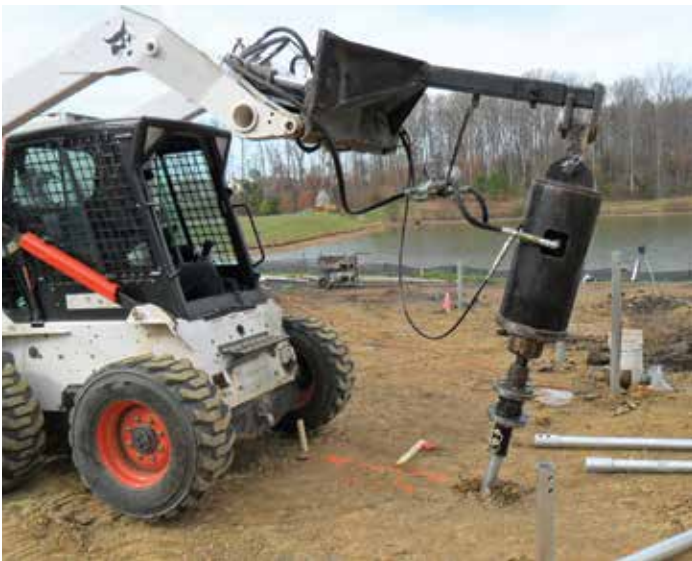
Machine-mounted drive head with bail assembly installing battered pile
