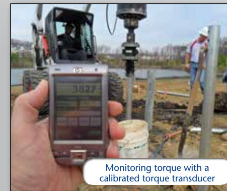
Lead section advanced at a 14-degree batter
