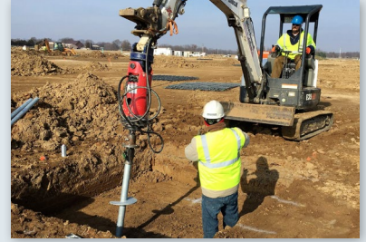
Installing battered lead section
