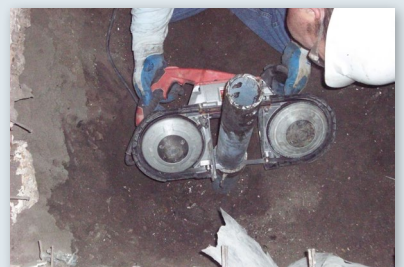
Cutting installed pile to specified elevation
