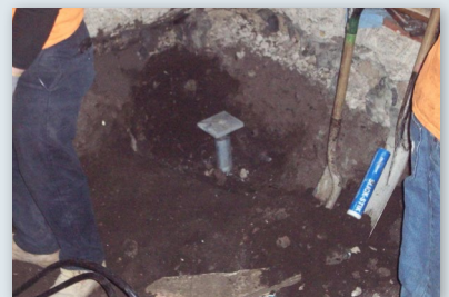
Helical pile installed and fitted with new construction cap
