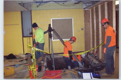
Installing helical piles with hand held equipment within proposed elevator pit
