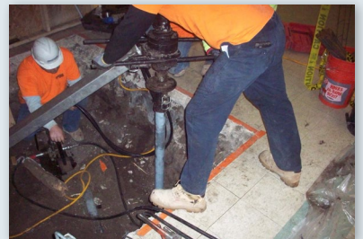
Advancing helical pile within pit excavation
