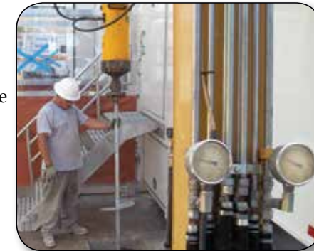
Figure 1: Dual pressure gauges mounted to arm of excavator
