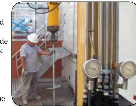
Figure 1: Dual pressure gauges mounted to arm of excavator
