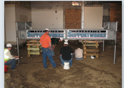
Load test completed and design capacities confirmed
