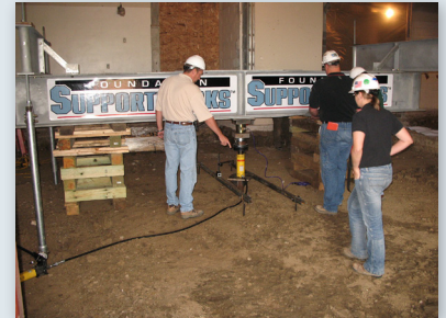
Load test set up prior to installation of performance piles
