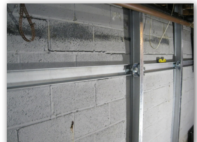
Cross-beam support on south wall
