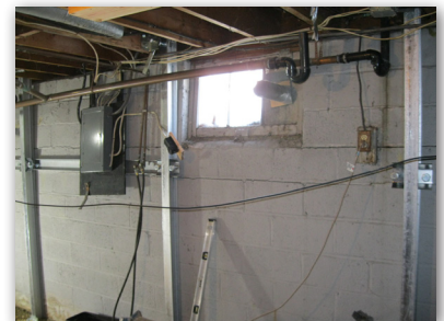
Installation around wall obstacles
