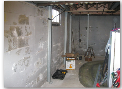
PowerBrace™ installed along north and west wall
