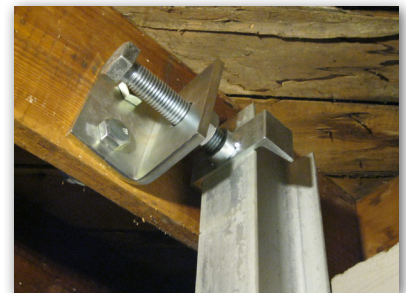
PowerBrace™ secured to floor joist
