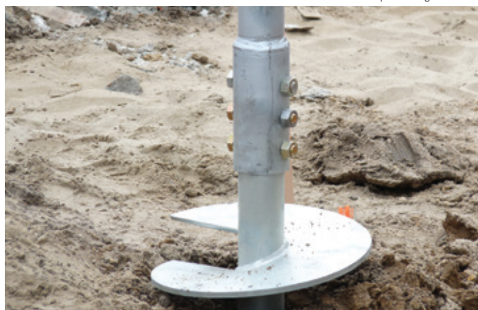
Galvanized helical pile being installed.
