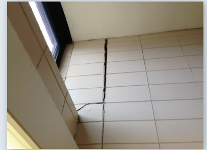
Cracks observed in CMU partition walls
