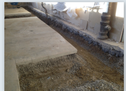
Demolition completed for pile installation
