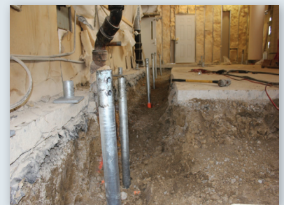
Installed piles to be cut to design elevation
