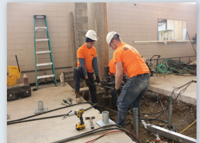
Helical piles installed with hand held equipment
