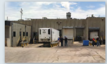
Existing loading docks
