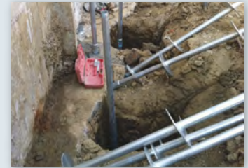
Leads and first extensions staged near installed piles
