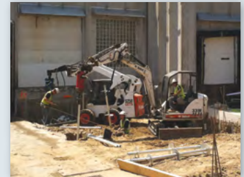
Skid-steer and mini-excavator installing helical piles
