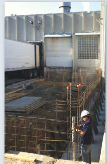
Setting pile elevations within columns and grade beams
