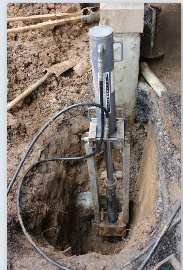
Advancing push piers to bedrock
