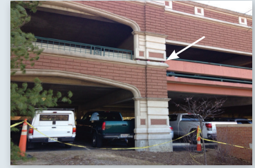
Settled façade; separation
