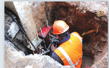
Connecting hydraulic lift cylinders
