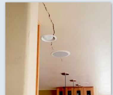
Drywall crack in ceiling (before)
