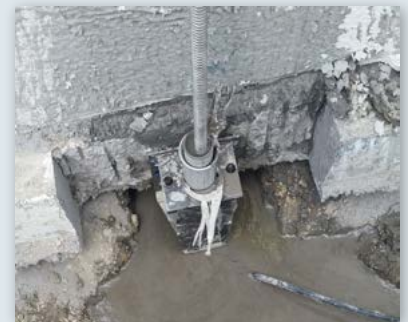
Grout-filled hole and pier tube
