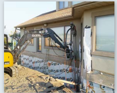
Drilling at micropile location
