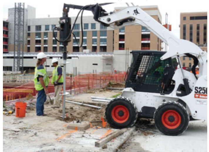
Helical piles to support crane pads at a construction site
