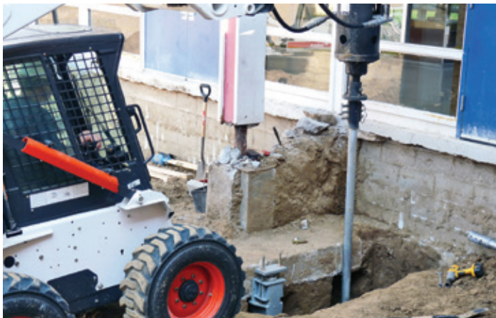
Retrofit helical piles to support an existing column at a school
