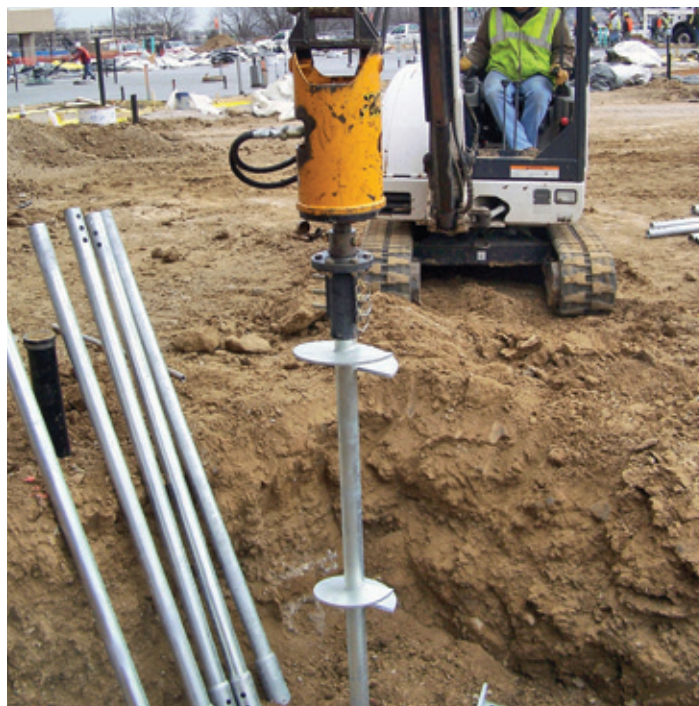
Helical piles to support foundations of a medical center addition
