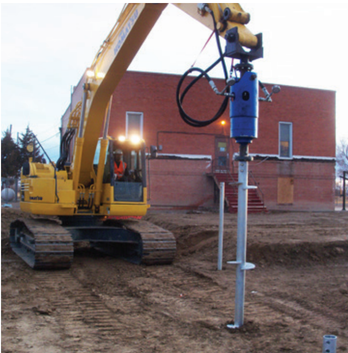
Helical piles to support foundations of a school addition
