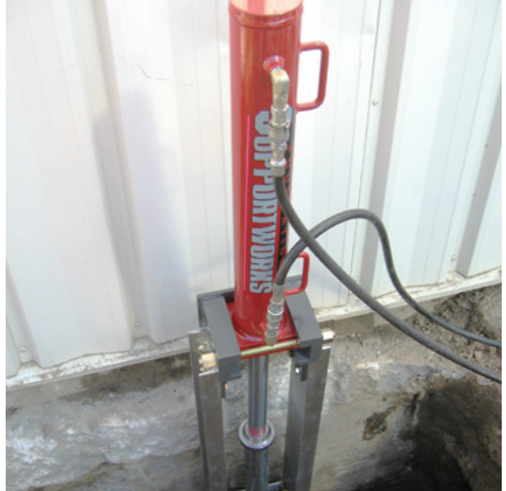
Hydraulic cylinder installing a 2-7/8 inch push pier.
