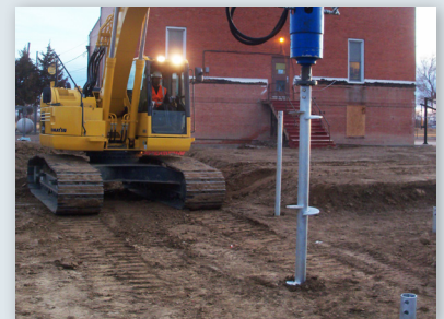
Installing HP450 helical pile
