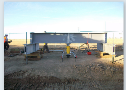
Helical pile load test
