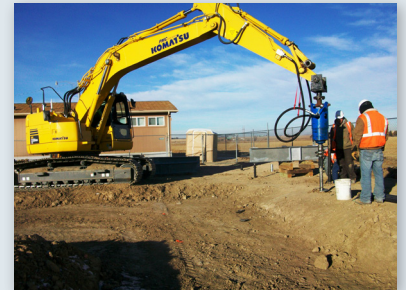
Installing test and reaction piles
