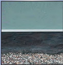
After - Installation of new Reinforced Perimeter Flashing Strip with butyl tape attached and EPDM flashing. New EPDM flashings are seamed to the underside of the existing EPDM field membrane.
