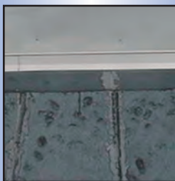
Before - Open seams and deteriorated surface on modified bitumen membrane on sloped wall
