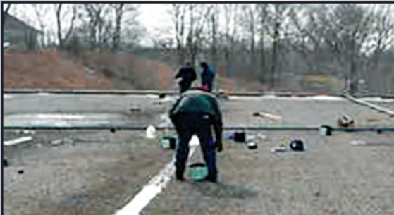
Repair of split membrane by using a three course flashing repair method, consisting of a base layer of plastic cement, a layer of asphalt coated fabric and a top layer of plastic cement.
